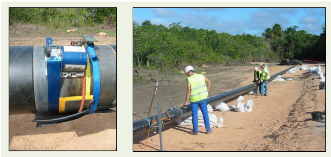
Figures 1 and 2. – The \gamma -Prox (contact version) in control situation on a 10'' pipe yard in French Guyana.
