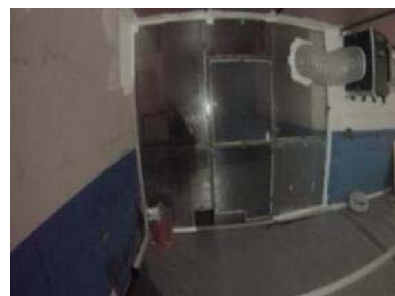
Partition door between internal containment and central part of the bunker
